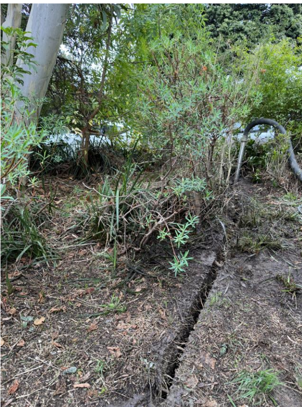
Figure 25 NDRI trench along proposed basement ramp in relation to tree 4
