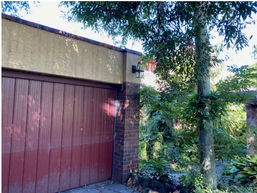
Figure 3 Detail of front façade showing the modern steel door cladding profile, rough cast, clinker brickwork, and a possible reproduction lamp
