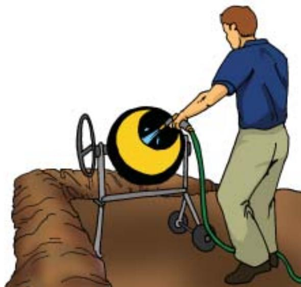
concrete slurry by tipping small amounts in a ditch lined with plastic or geotextile liners. When the water evaporates or soaks into the surface the solids can then be put into a skip bin or recycled in construction or as road base.
