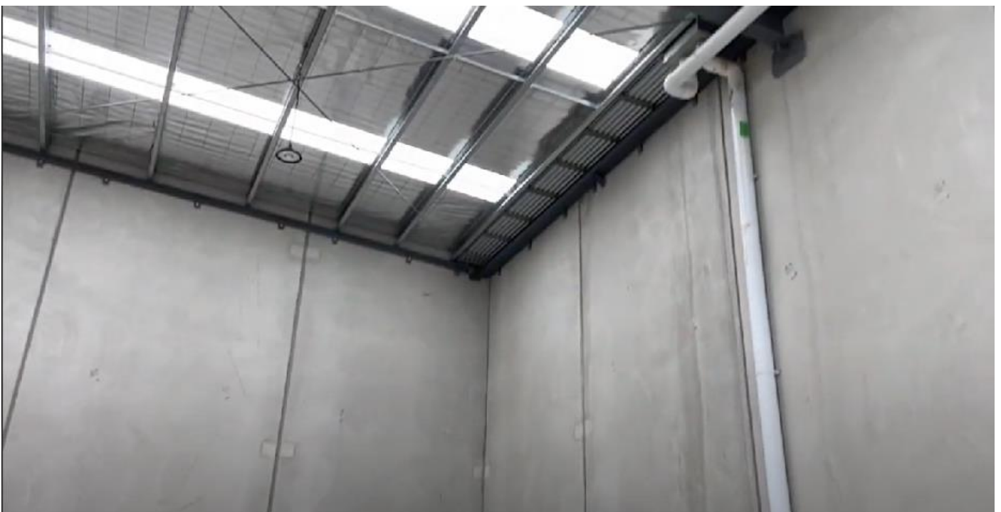
Tilt slab walls and roof construction within the site.
