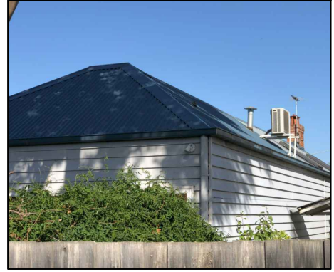
EXISTING ROOF & BOUNDARY WALL
