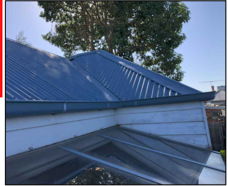
EXISTING ROOF & SKYLIGHT
