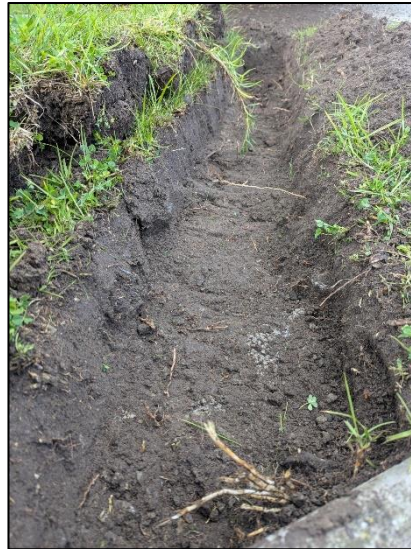
Open trench to ~400mm depth
